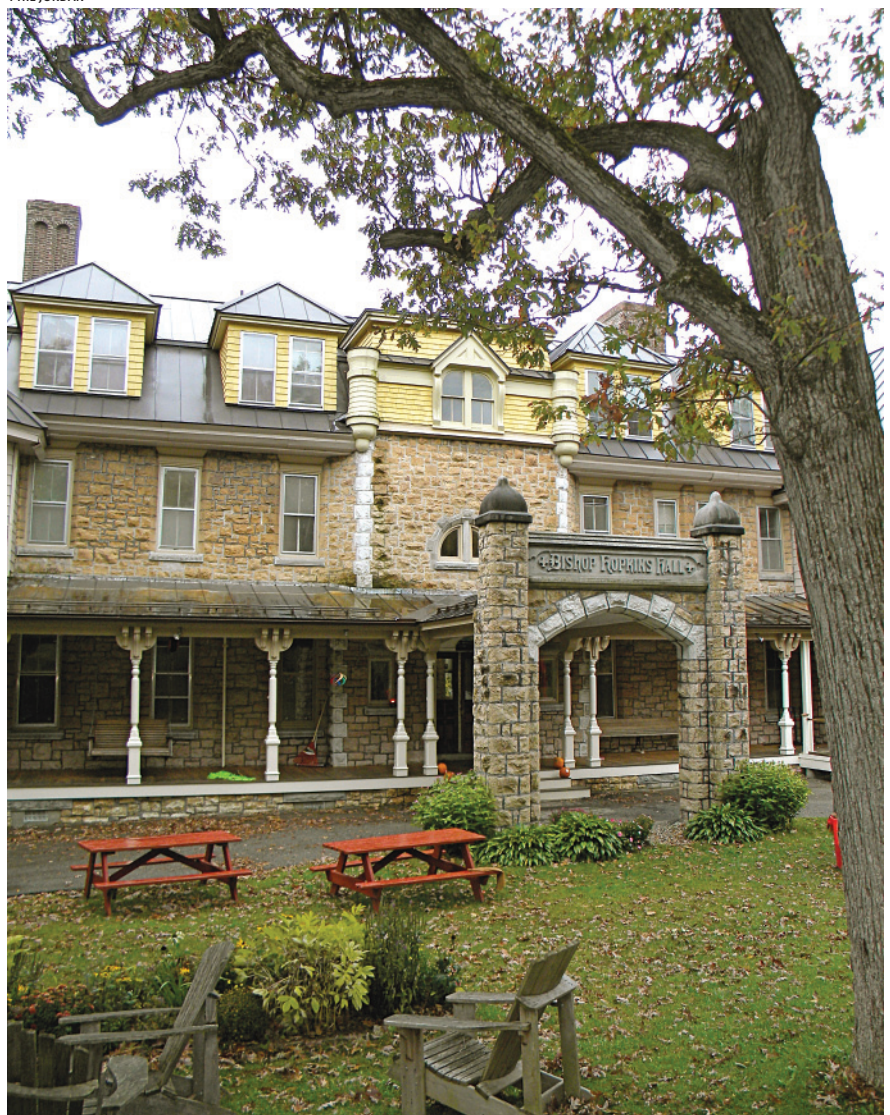
The portico of Rock Point School's stately main building, built in 1888, still bears the name of the finishing school that preceded it, Bishop Hopkins Hall. The building is owned by the Episcopal Church but operated by Rock Point School.
